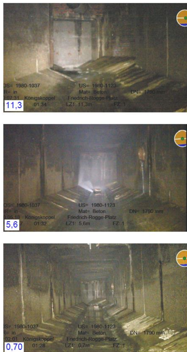
Figure 1. TV-inspection frame before the rehabilitation
