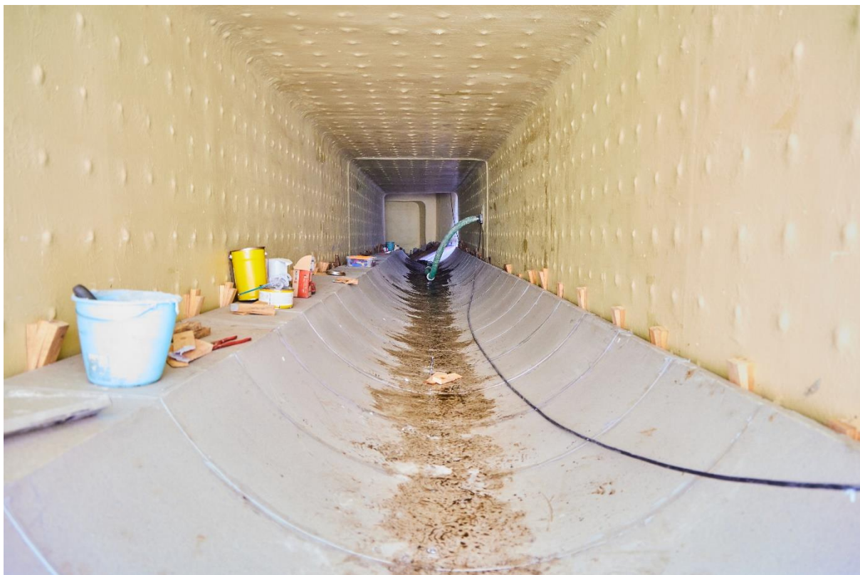
Figure 8. Installation of the panels
